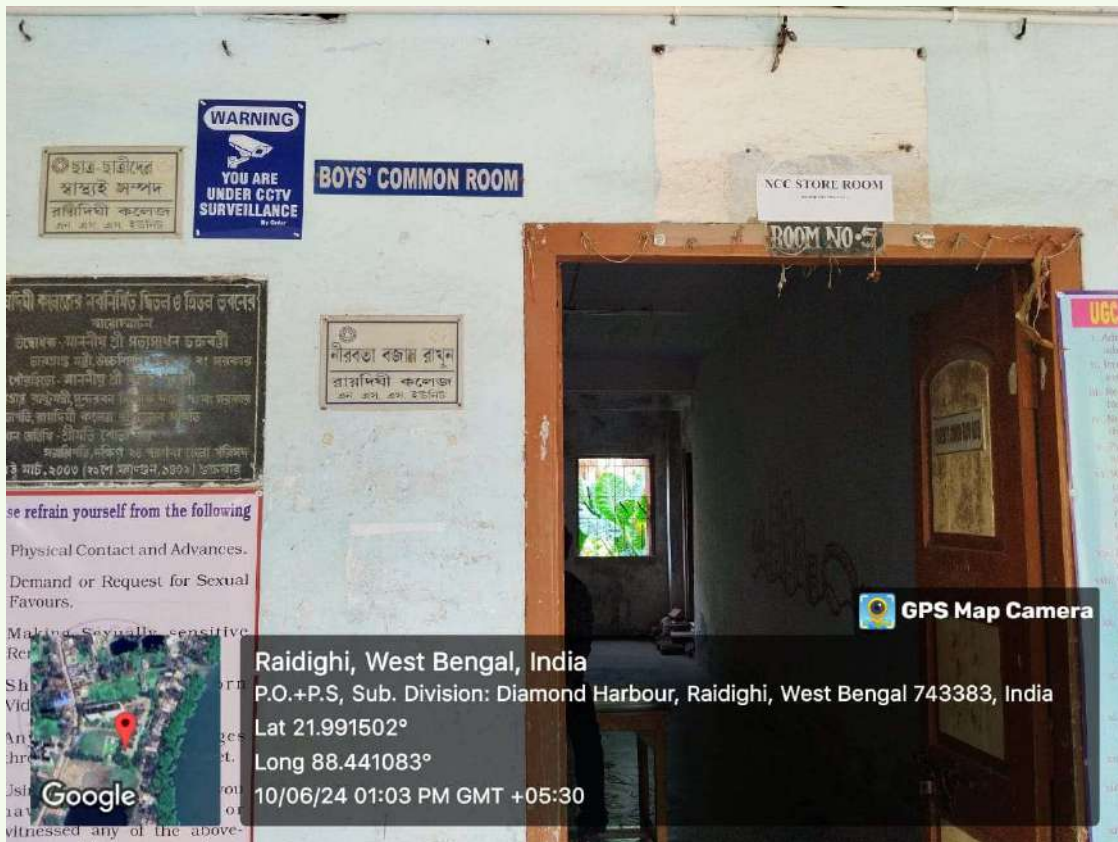
BOYS' COMMON ROOM: FRONT VIEW
