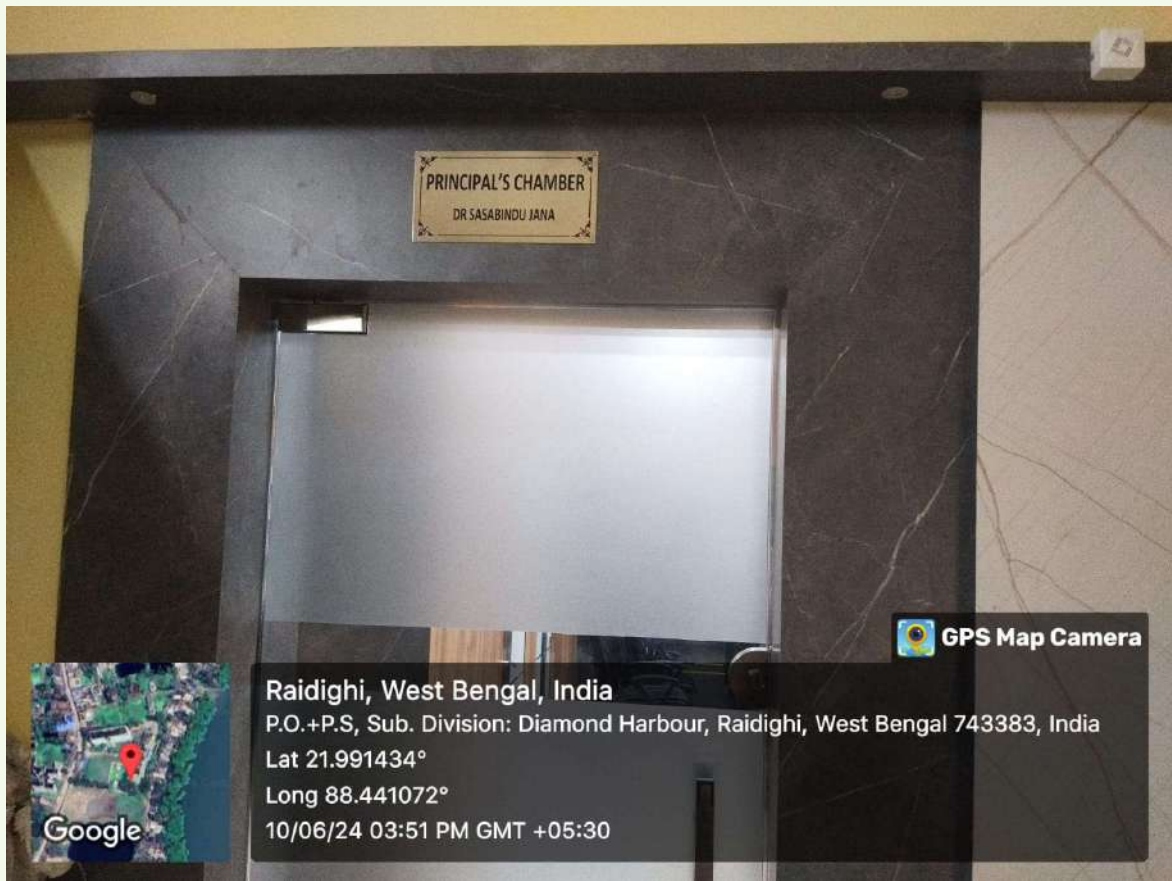
PRINCIPAL CHAMBER: FRONT VIEW
